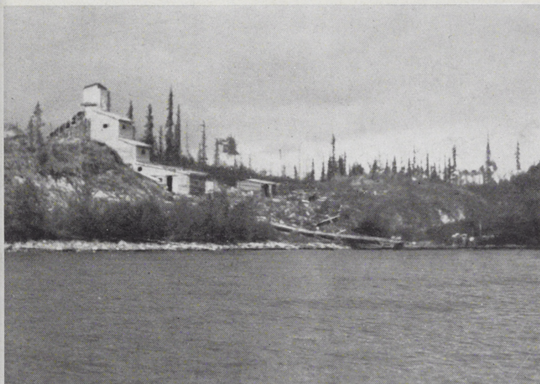
Pilot testing mill of De Staffany Tantalum Beryllium Mines Limited. First unit of plant to treat Tantalum and Columbium Ores—the wonder metals of the new age. The mill treats 25 tons of ore daily.
